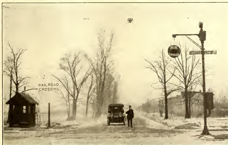
NORTH SHORE GRADE-CROSSING PROTECTION—AUTOMATIC WIG-WAG SIGNAL AND SIGN INSTALLED AT CROSSING AND WARNING SIGNAL INSTALLED 300 FT. AWAY
